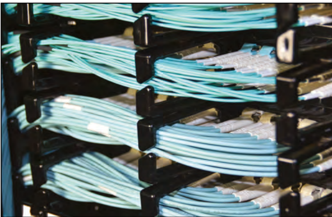
High Density LC Patching in the RapidNet Distribution Chassis
