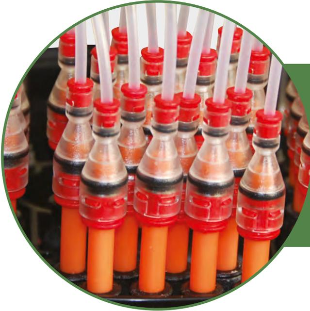
The blown fibre tubing that enters the closure through the ports are all fitted with reducers as standard. These reducers produce a seal between the blown fibre tubing and the transportation tubing, allowing the fibre to be blown up into the closures and directly onto the fibre splice trays.
